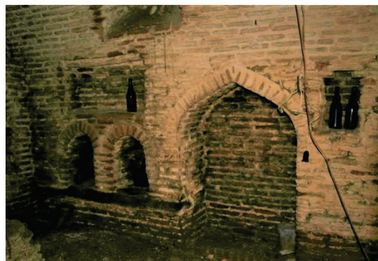
Fig. 2. A spacious cellar's wall with niches, 17th century. 21 G. Abesadze Str.
